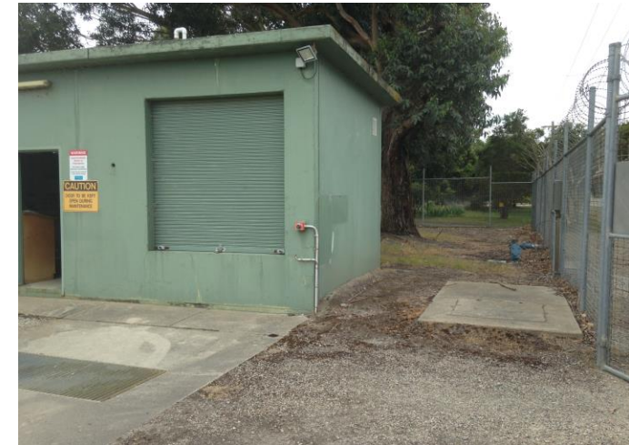
Chlorinator building with s. hypo storage inside
